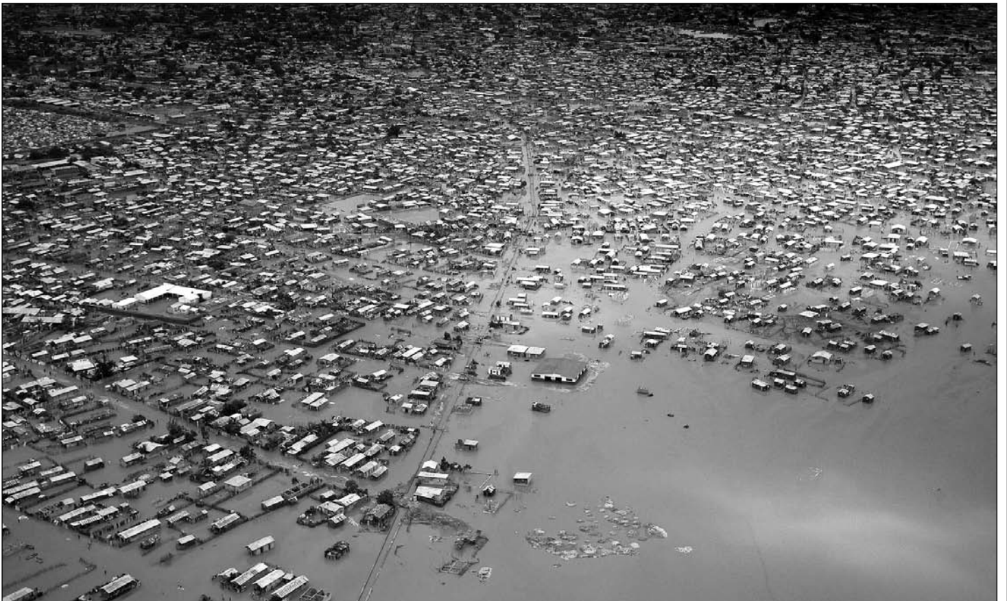
A city under water - Gonaïves, September 2008
