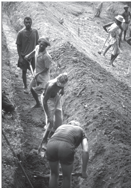
Anglo-Haitian 'konbit' (work brigade) digging anti-soil erosion ditches.
